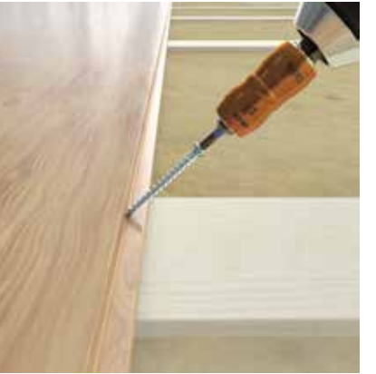
Floorboard assembly
